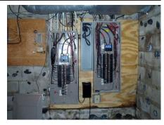
Maximum Capacity: 200 AmpsAcceptableMain Breaker Size: 200 AmpsAcceptableBreakers: Copper and AluminumIs the panel bonded? NoUpper bedroom closet Electric Panel
