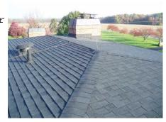
Type: Gable Approximate Age: 10-15 years Mansard sides Roof Surface -Method of Inspection: Ground level
