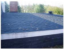
Type: Gable Approximate Age: 10-15 years Main Roof Surface -Method of Inspection: Walked on the roof
